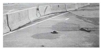
Fig. 2. Concrete barrier displacement on impact of a vehicle [2]
